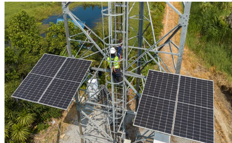
→ Solar Power Installation at Cell Site
